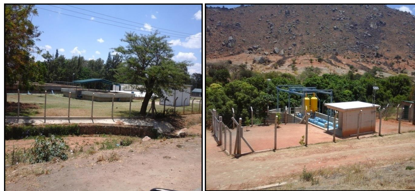
Plate 7.1: Intake structure and conventional treatment plant at Ndiuka
