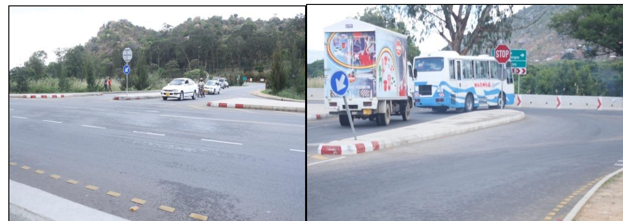
TAMZAM highway, showing tarmac road
