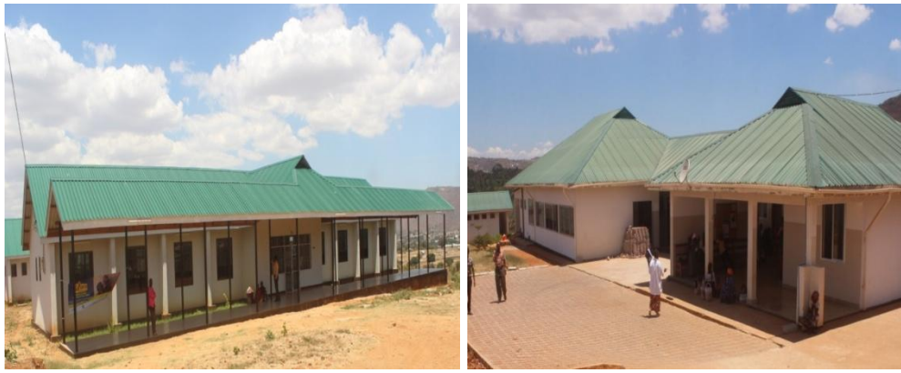
Frelimo Hospital Maternity block and OPD
